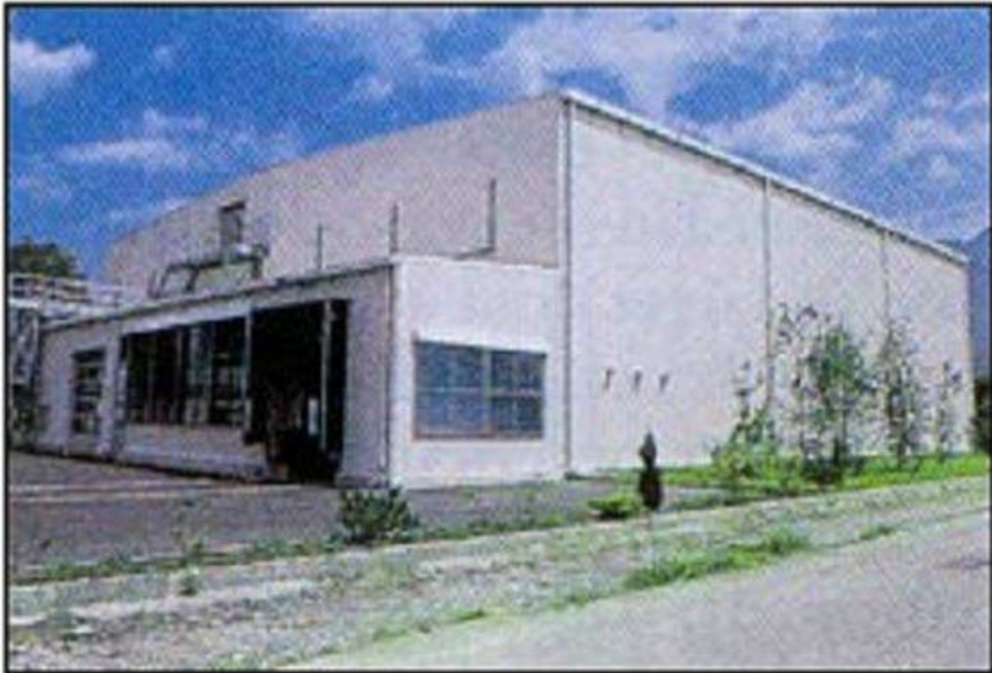
Large size cold storage made of PUF panels
